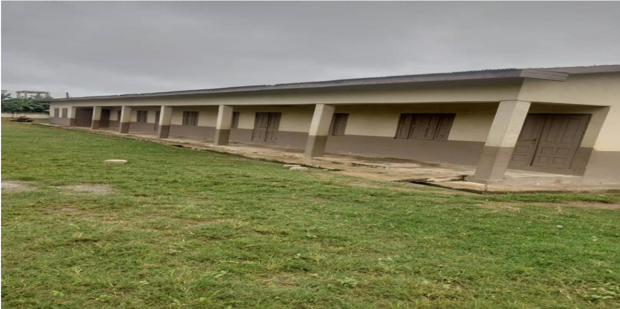
Constructed 1no 3unit Classroom Block at Jamasi
