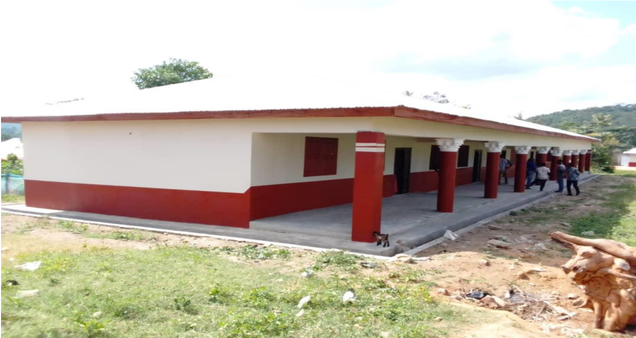
Constructed 1no 3unit Classroom Block at Bepose
